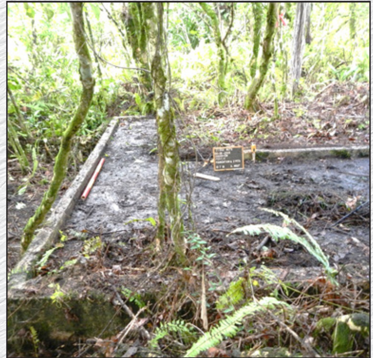
Concrete foundation for Quonset hut
